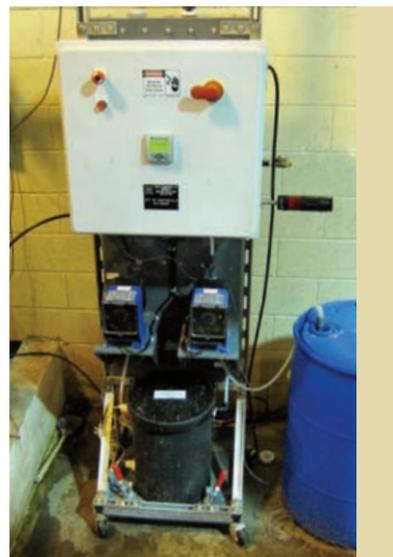
The chlorine dioxide generator is located at the head of the plant. At left is a corner of the influent trough that is dosed with the compound.
